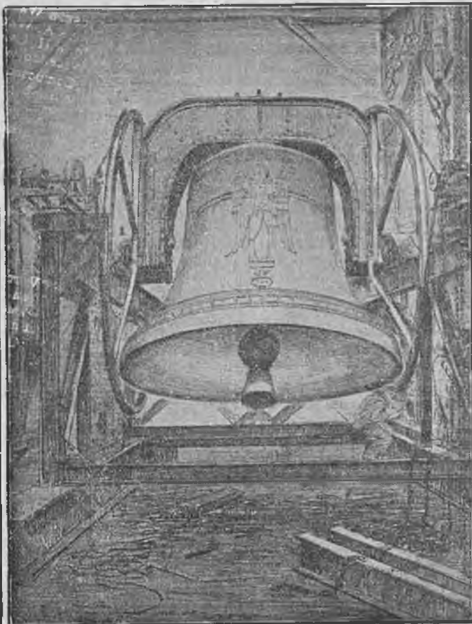
THE 18½ TON RINGING BELL, the Bourdon of the Carillon of 64 Bells, about to be installed at RIVERSIDE CHURCH, NEW YORK, U.S.A.
