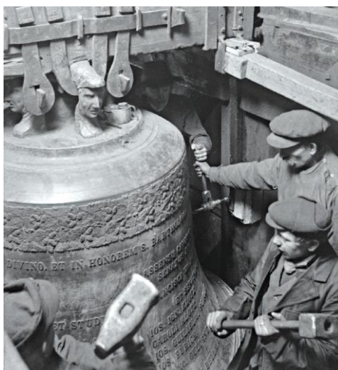
Getting ready to break a bell at Plzni in the Czech Republic in 1917 so the metal can be easily removed
