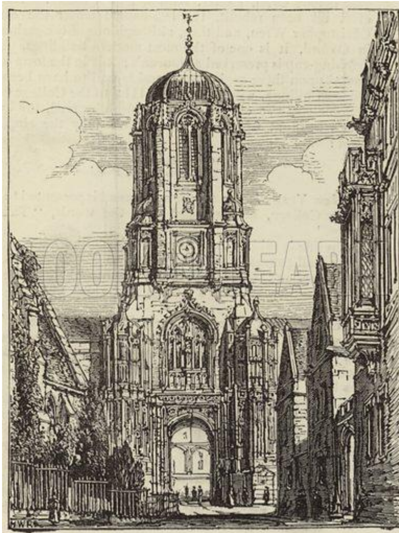
Print of the gate house and tower
