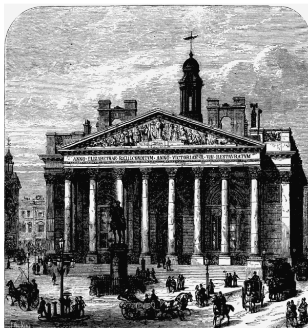
The present Royal Exchange building
