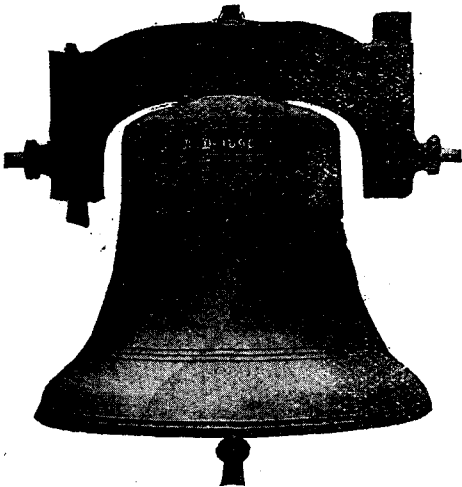
New Tenor Bell, St. Paul's Church, Bedford.
